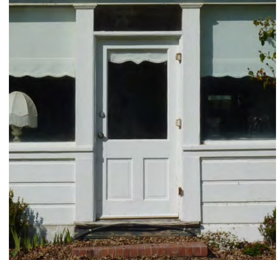
Figure 75. Single lite over two-panel door at sunroom.
