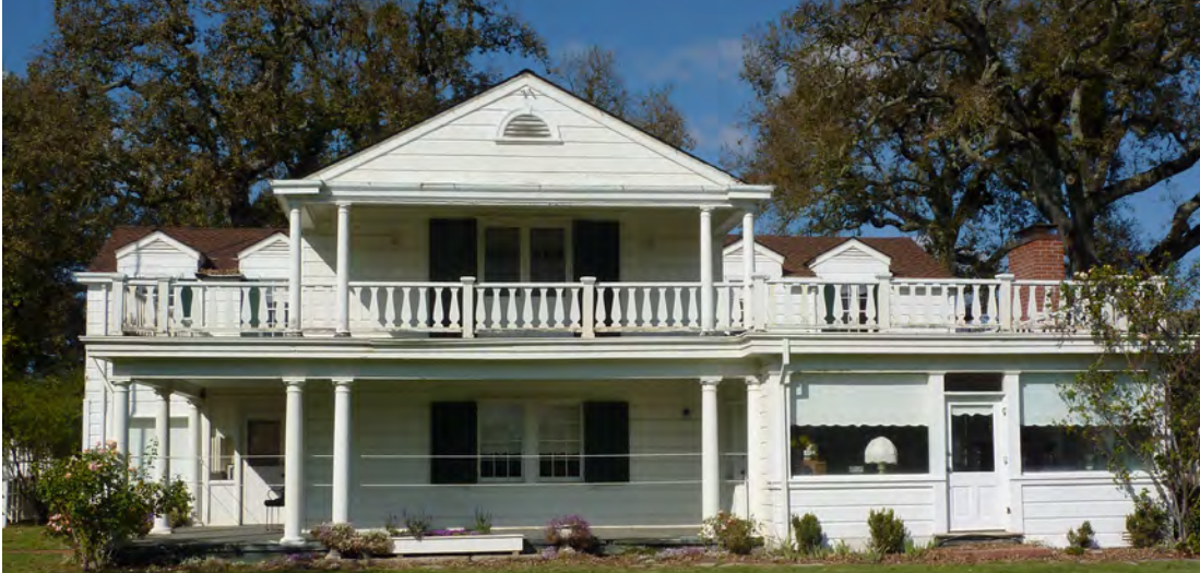
Figure 30. Southeast Elevation of Main House.
