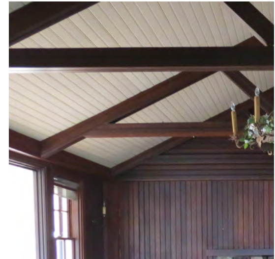
Figure 182. Sloped bead board ceiling in Room 102 with exposed timber rafters.
