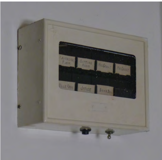
Figure 256. Push-bell enunciator system.
