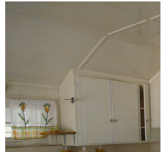
Figure 302. Battens at seams of gypsum board.
