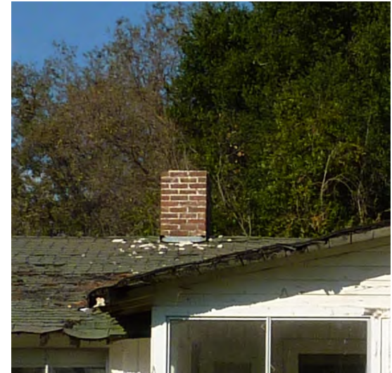
Figure 325. Brick interior chimney.
