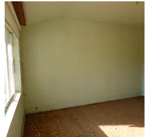
Figure 342. Typical gypsum board wall found throughout McCreery Cottage.
