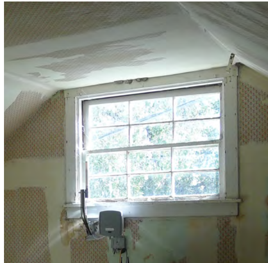
Figure 305. Flat wood trim surrounding window.
