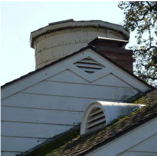
Figure 157. Painted louvered attic vents.
