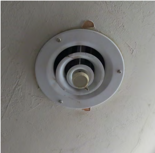
Figure 255. Circular ceiling-mounted diffuser.
