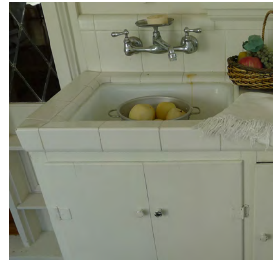
Figure 117. Non-contributing under mounted kitchen sink.
