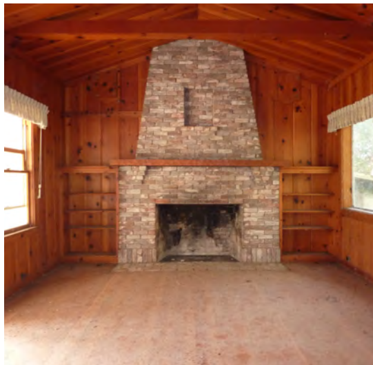
Figure 350. Brick fireplace in Living Room.
