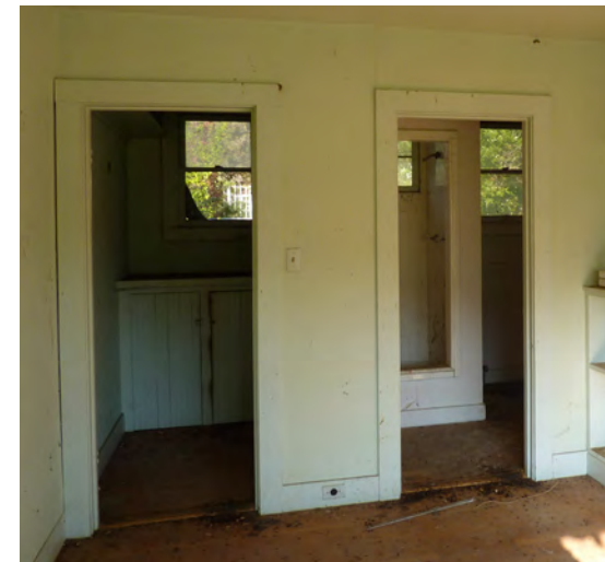
Figure 346. Flat trim around door openings.
