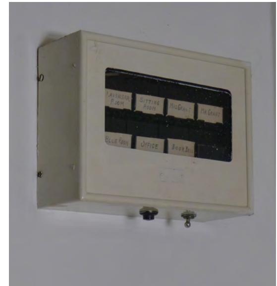
Figure 124. Push bell enunciator in Maid’s Room.
