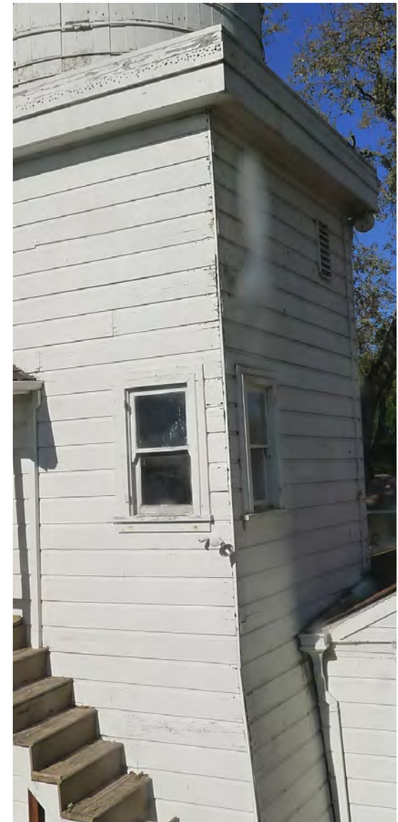
Figure 135. Double hung wood windows on northeast and southeast elevations.
