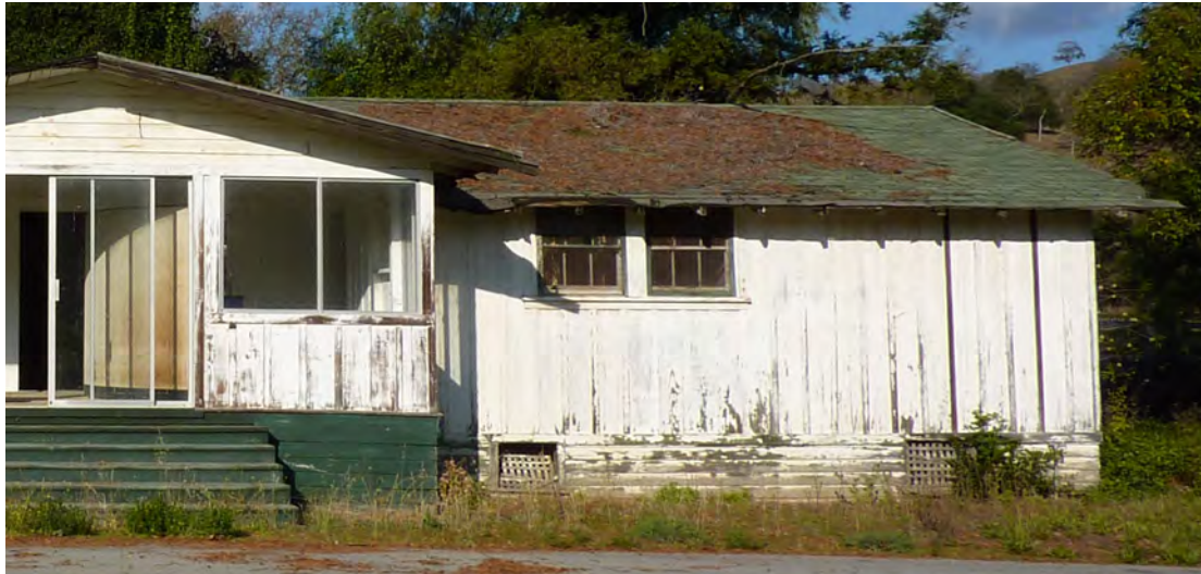
Figure 327. Board and batten siding above shiplap siding on McCreery Cottage.
