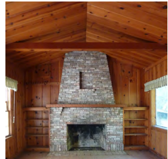
Figure 315. View of brick fireplace in Room 102 - Living Room.
