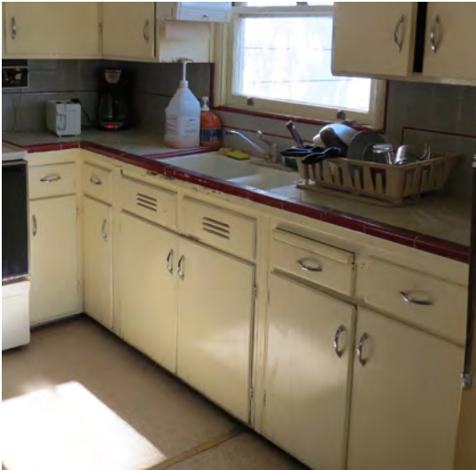
Figure 249. Built-in kitchen cabinetry with tile countertop.
