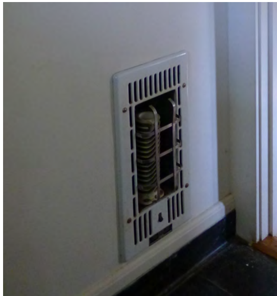
Figure 122. Typical bathroom electrical heater.
