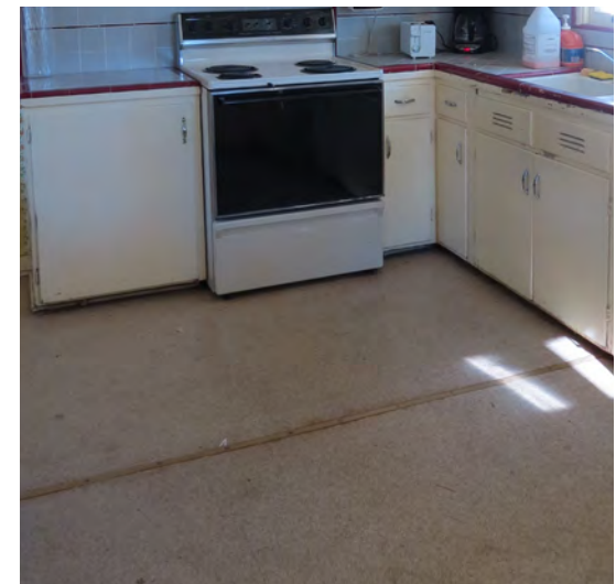
Figure 240. Vinyl floor in Room 102 - Kitchen.
