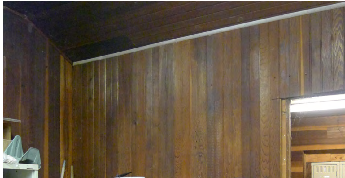
Figure 242. Bead board walls in Room 105 - Original wood shed.
