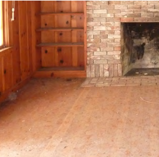
Figure 338. Wood floor in Living Room.
