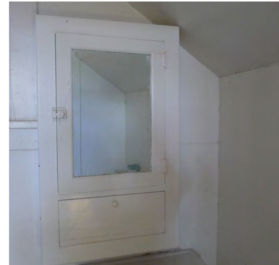
Figure 306. Wood medicine cabinet in Room 202.
