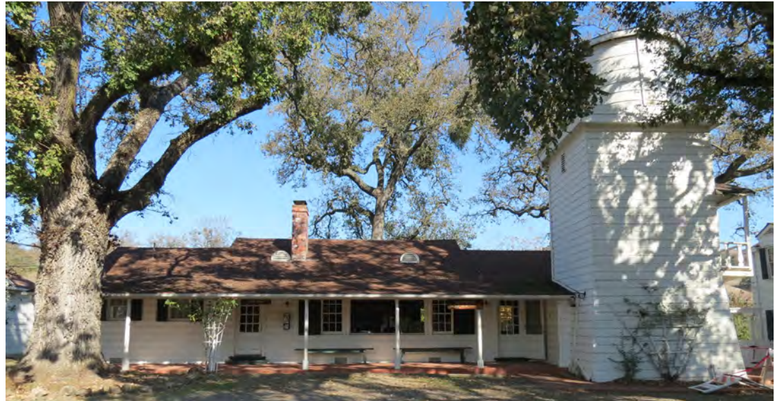
Figure 144. Southwest Elevation of Cook House.
