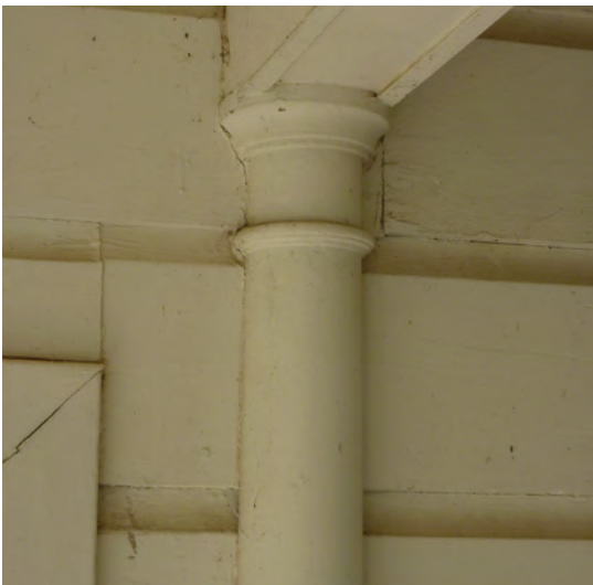
Figure 279. Engaged column.
