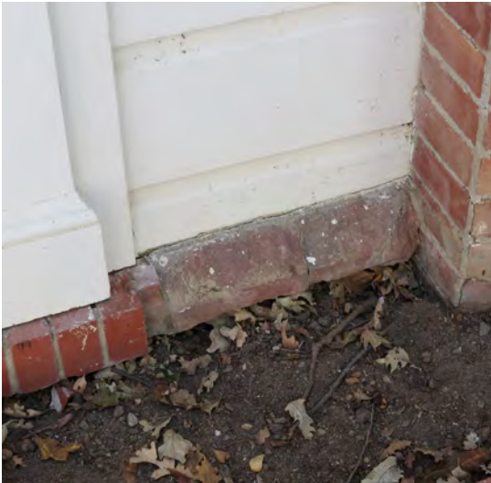
Figure 87. Small exposed section of brick clad foundation.
