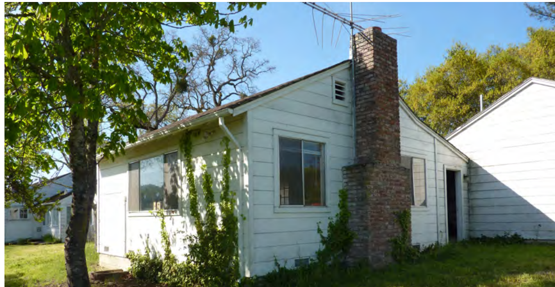
Figure 201. View of 1960s addition from north.
