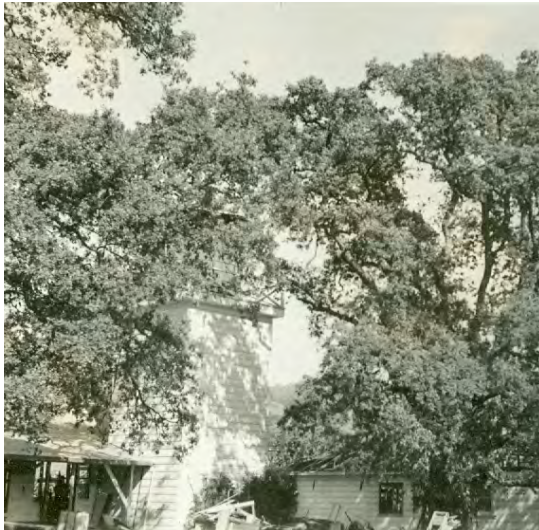
Figure 22. Complex under construction, 1937 (Grant Park Archives).
