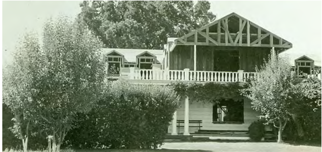
Figure 23. Main House under construction, c.1937 (Grant Park Archives).
