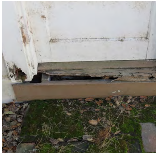
Figure 233. Heavy biological growth on brick step.
