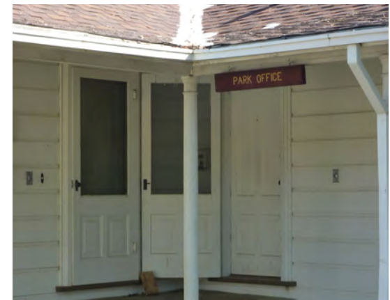
Figure 222. Four-panel wood doors with screens.
