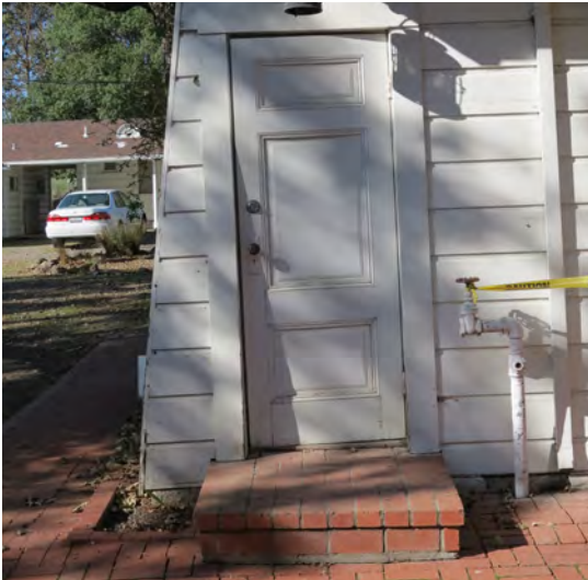
Figure 133. Three-panel wood door at first floor.
