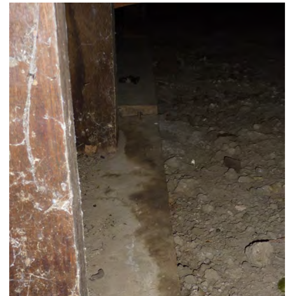
Figure 332. Perimeter stud wall at foundation.
