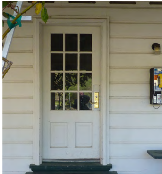
Figure 166. 12-lite over two-panel wood door on southwest elevation.
