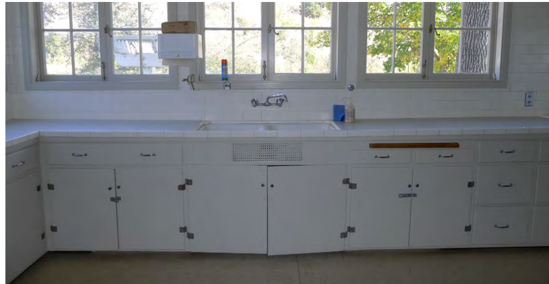
Figure 186. Under-counter cabinets in Room 104.
