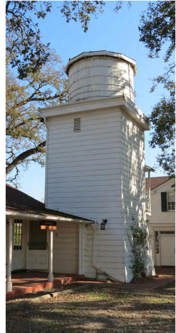
Figure 125. View of Tank House from west.
