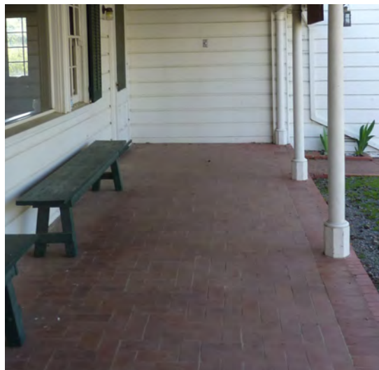
Figure 172. Brick breezeway in good condition.
