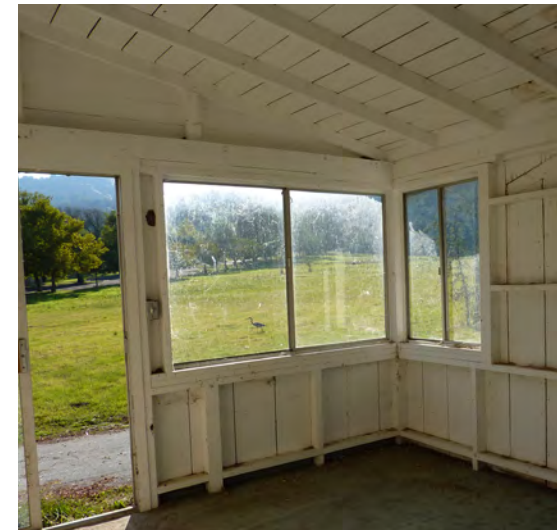
Figure 314. Room 101 - Enclosed porch.
