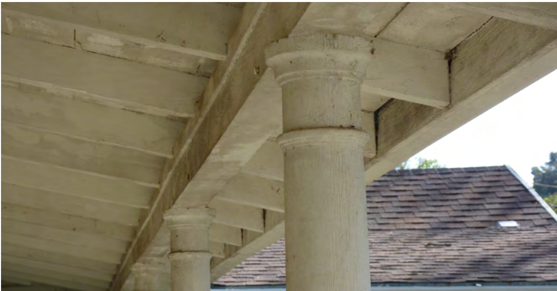
Figure 227. Wood columns at covered porch.
