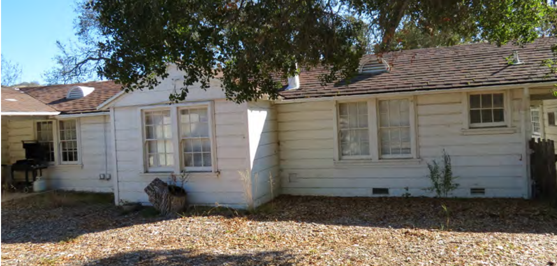
Figure 197. Northwest Elevation at courtyard.
