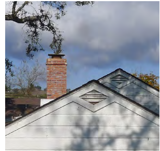
Figure 159. Brick interior chimney.
