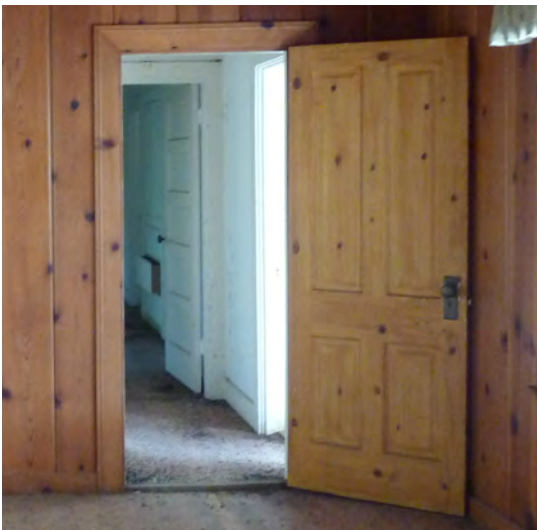
Figure 344. Four-panel door with five-panel door in the background.
