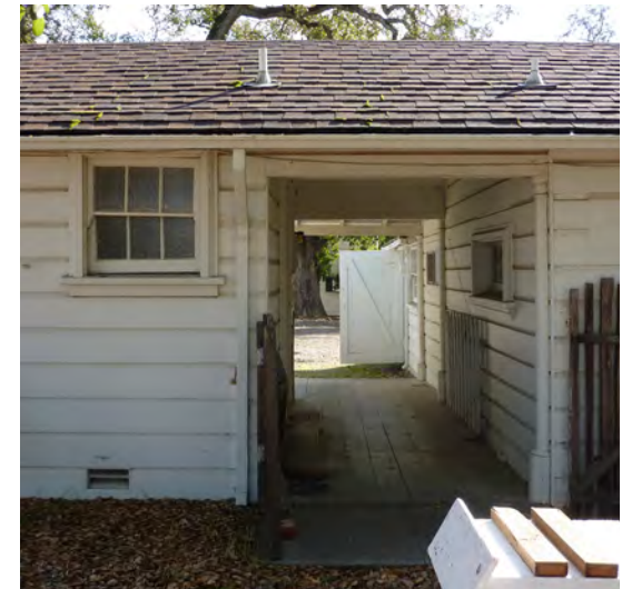
Figure 198. View of breezeway at Northwest Elevation.
