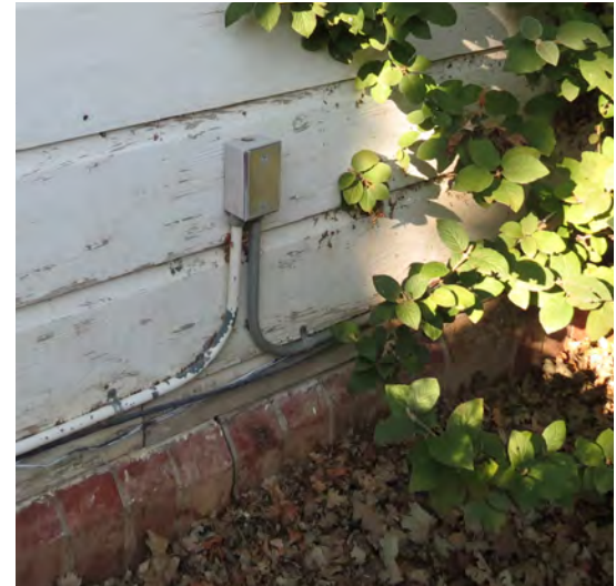
Figure 173. Brick with cracked mortar cladding concrete foundation.
