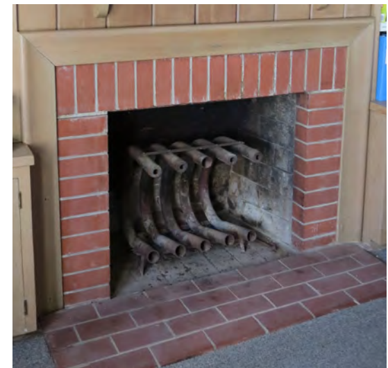
Figure 252. Brick fireplace in Room 103.
