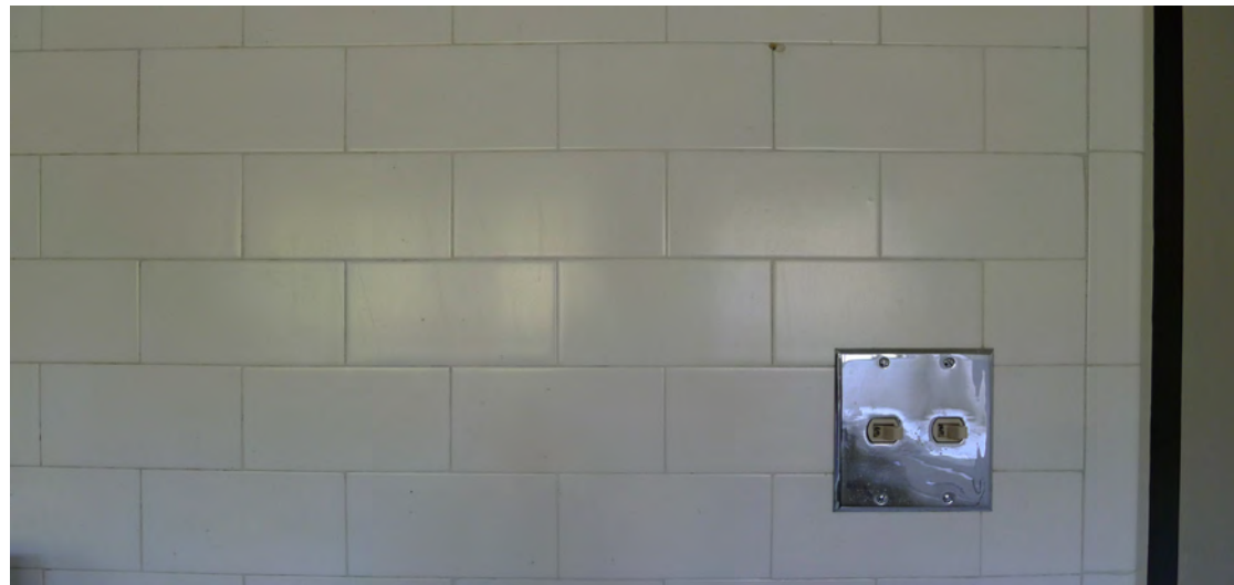
Figure 180. Subway tile in Room 104.
