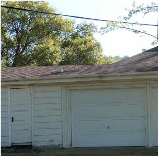
Figure 282. Five-panel door and metal garage door.
