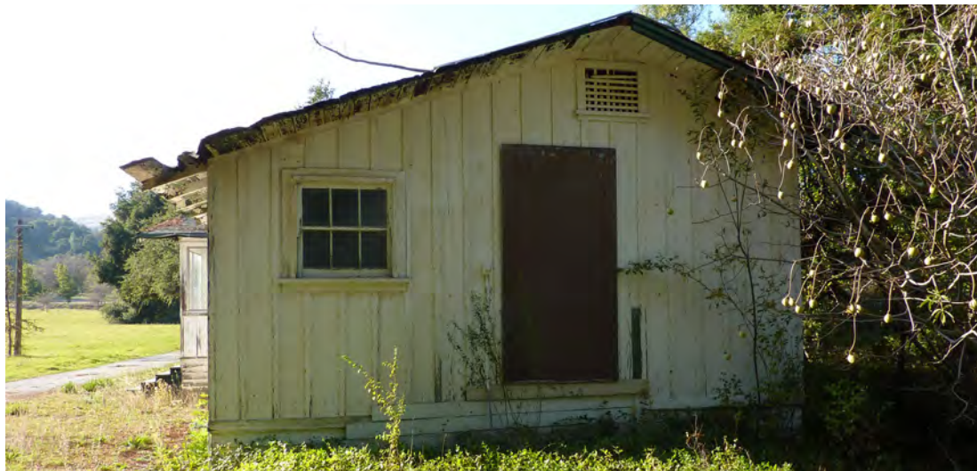
Figure 313. Southeast Elevation of McCreery Cottage.
