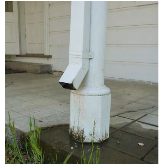
Figure 218. Downspout at base of wood column.
