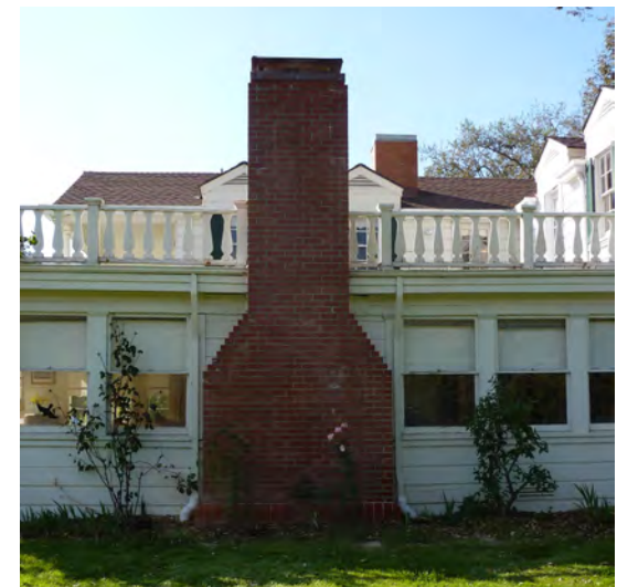
Figure 67. Brick chimney adjacent to Room 104 - Sunroom.
