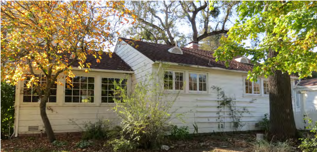
Figure 145. Northeast Elevation of Cook House.
