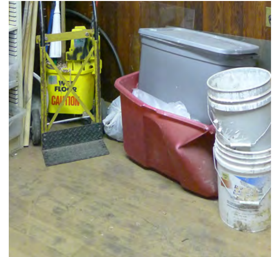
Figure 239. Wood floor in Room 105 - Original wood shed.
