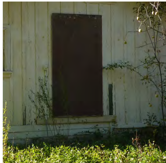
Figure 329. Boarded up door on east elevation.
