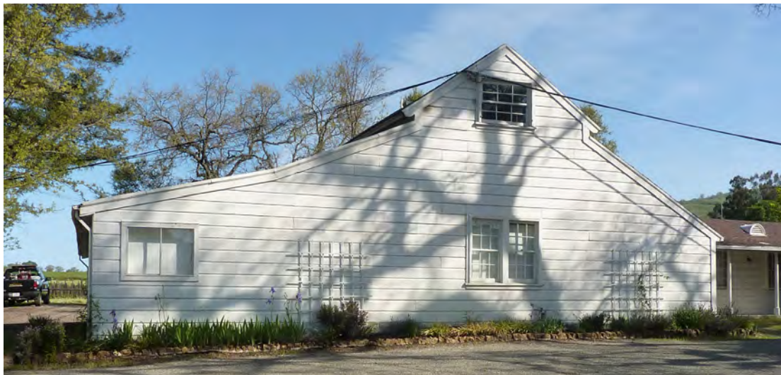
Figure 295. Trellises along the southwest elevation.
