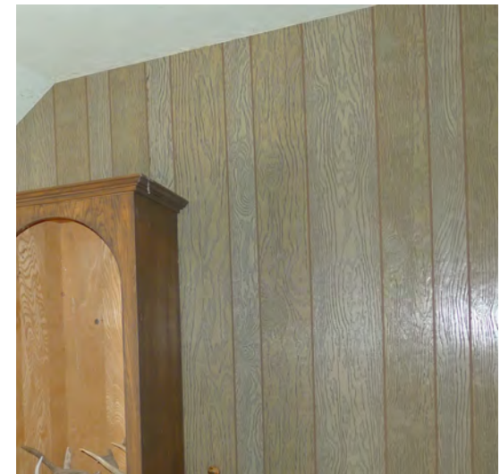
Figure 298. Wood veneer paneling.
