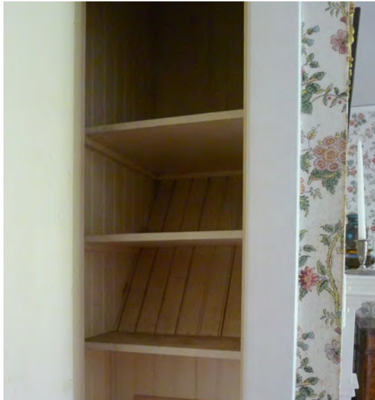
Figure 43. Room 105C - Closet mimicking chimney stack profile.
