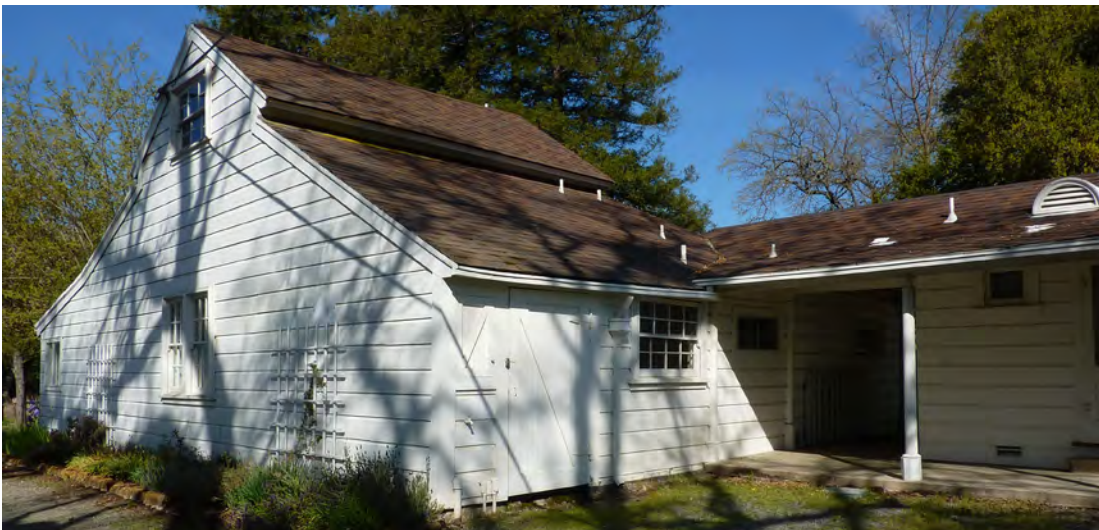
Figure 259. Northeast Elevation of Carriage House.
