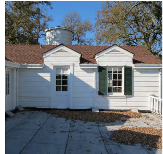
Figure 63. Roll roofing balcony floor.
