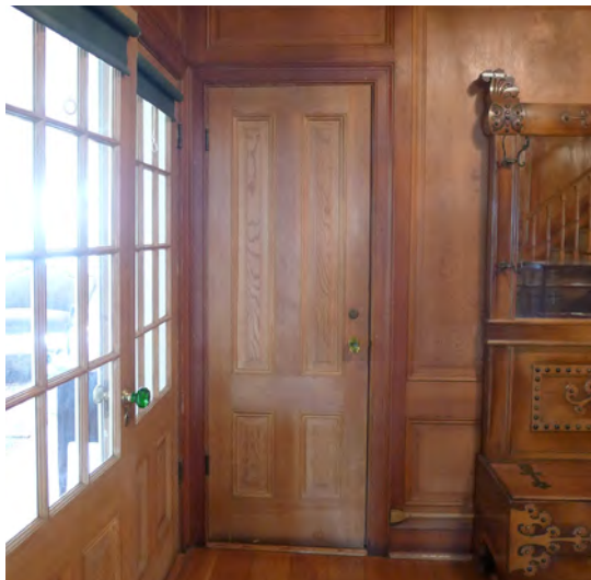
Figure 107. Four-panel wood door off Main Hall.
