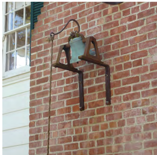
Figure 66. Brick chimney with attached bell.
