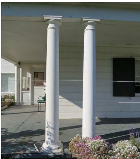
Figure 79. Pair of columns supporting second floor balcony.
