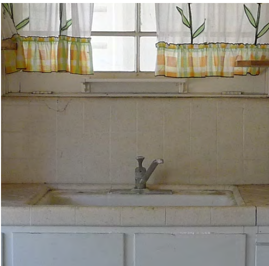
Figure 308. Ceramic sink installed during remodel.
