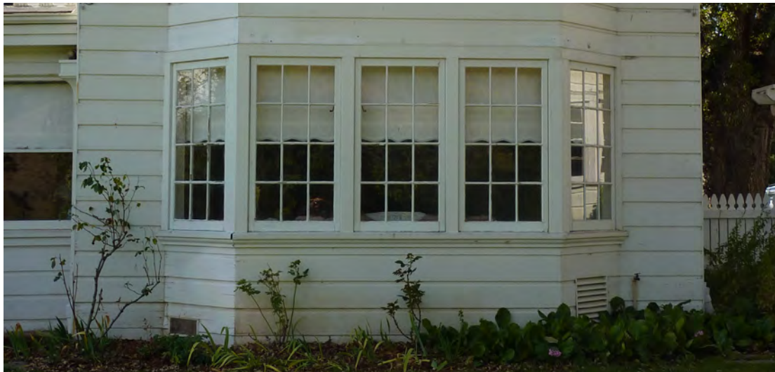
Figure 76. Multi-lite wood casement windows.
