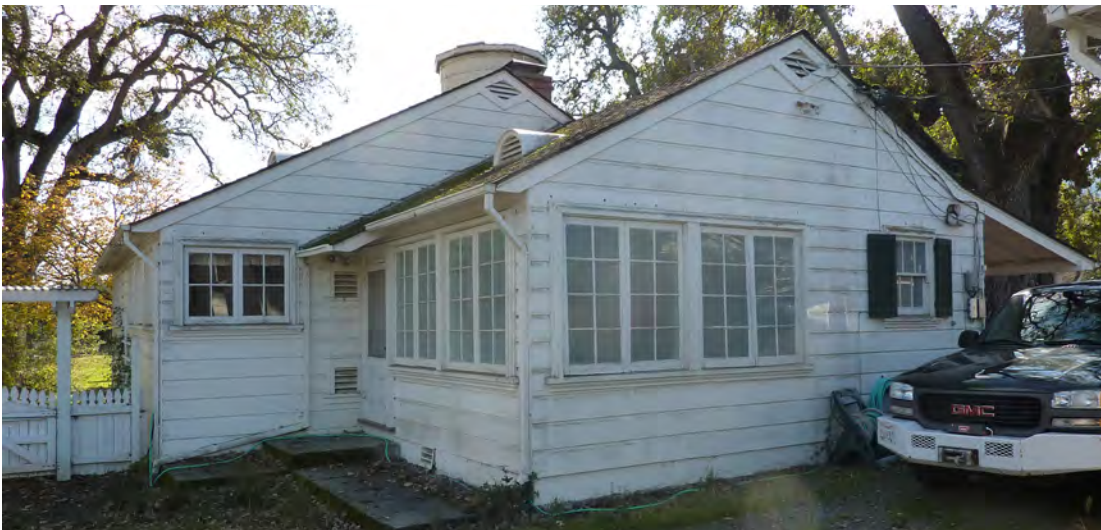
Figure 146. Northwest Elevation of Cook House.
