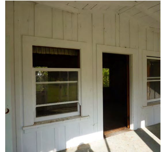
Figure 341. Board and batten wall finish at the Enclosed Porch.
