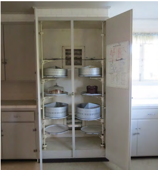
Figure 185. California Cooler in Room 104.
