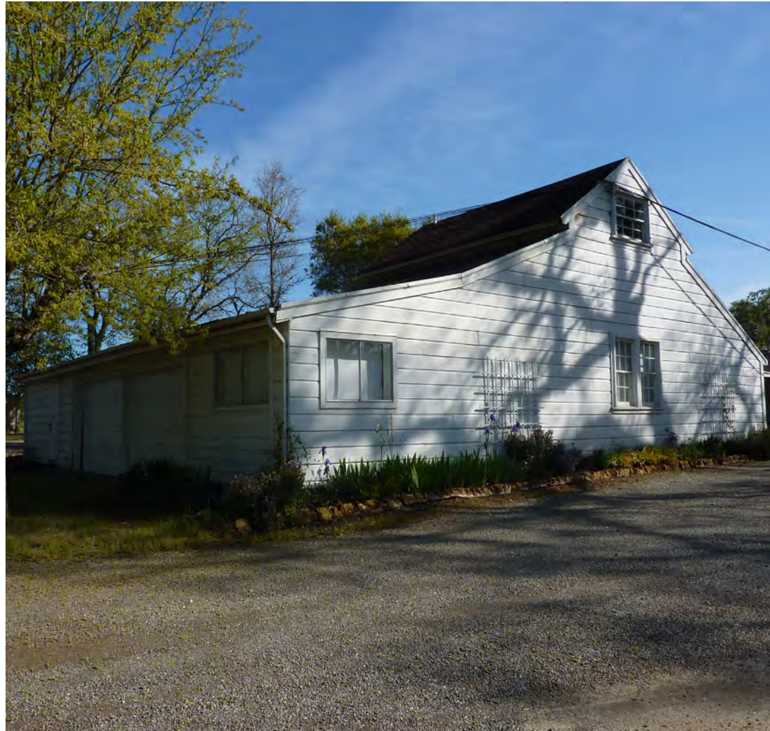
Figure 257. View of Carriage House from south.
