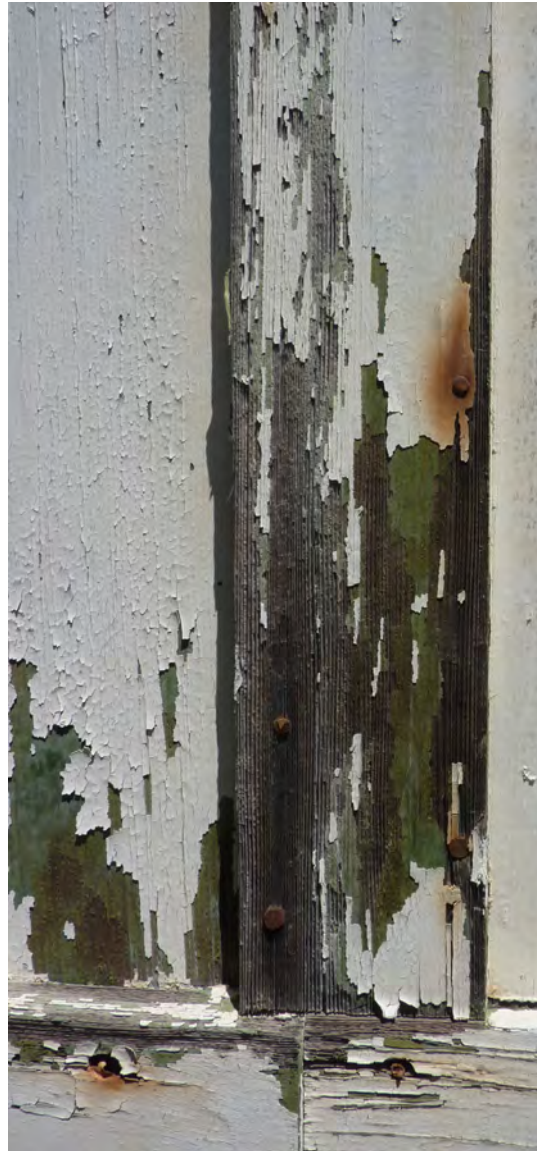
Figure 333. Peeling paint.
