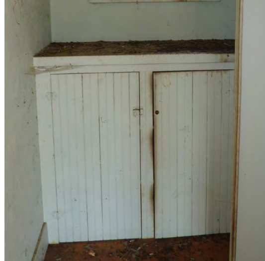
Figure 348. Cabinet in Room 106A.
