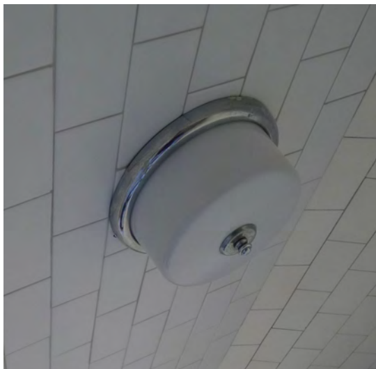
Figure 194. Original ceiling mounted light fixture in Room 104.
