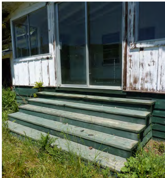
Figure 331. Wooden entry steps.
