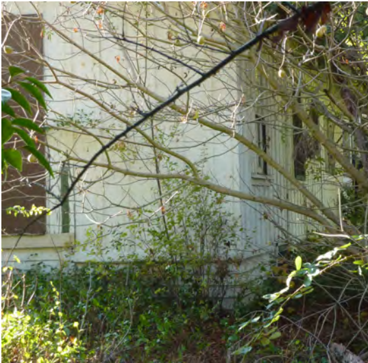
Figure 336. Vegetation close to McCreery Cottage along the northeast elevation.
