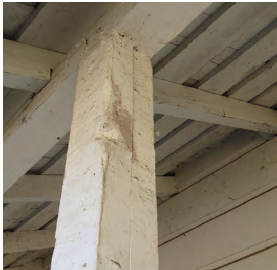
Figure 288. 2x4 wood studs used for post.
