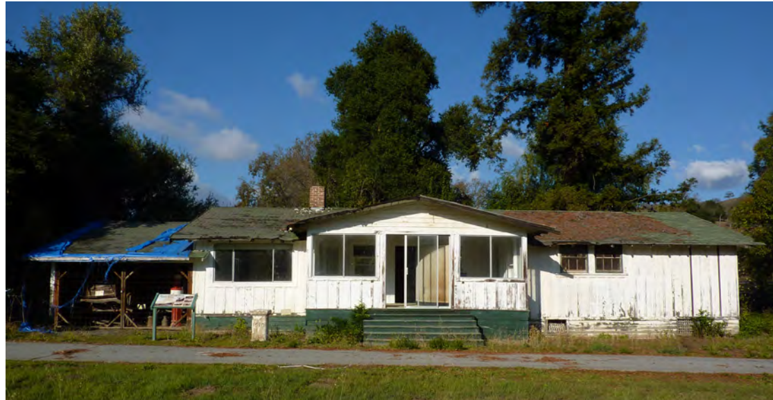
Figure 311. Southwest Elevation of McCreery Cottage.
