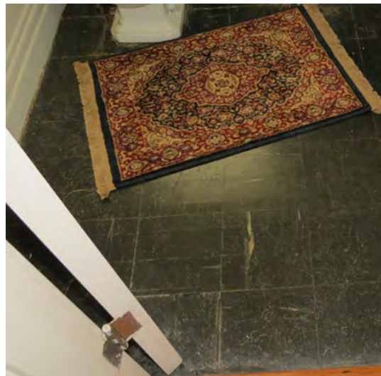
Figure 94. Non-contributing vinyl tile floor in Room 106.
