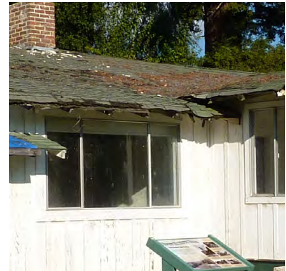
Figure 322. Deteriorated shingles.
