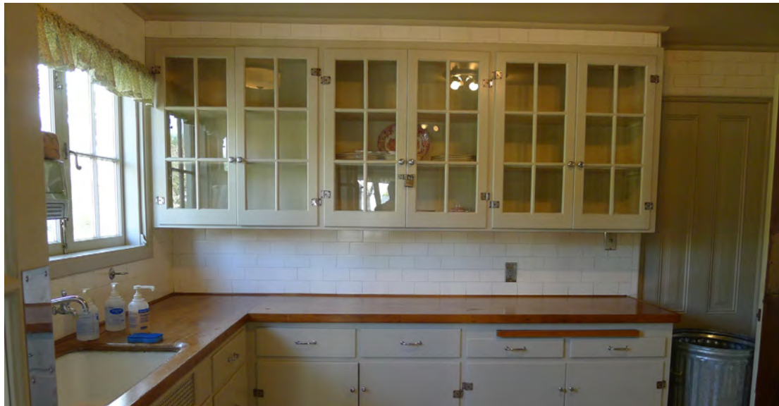
Figure 187. Wall-mounted cabinets with multi-lite glazed doors in Room 103.
