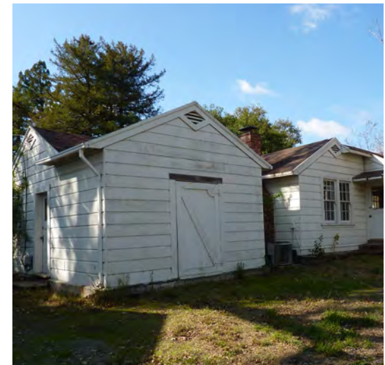
Figure 199. Partial Northeast Elevation.
