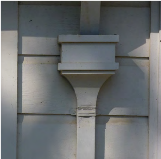
Figure 278. Decorative wood downspout cover.
