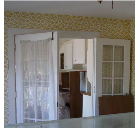
Figure 304. 10-lite wood doors surrounded by flat trim.
