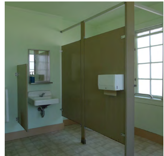
Figure 156. Room 108 - Men’s Bathroom.
