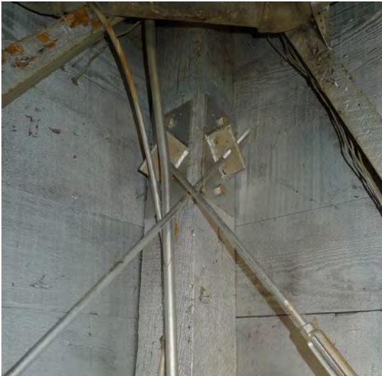
Figure 142. Diagonal ties and exposed wood framing.
