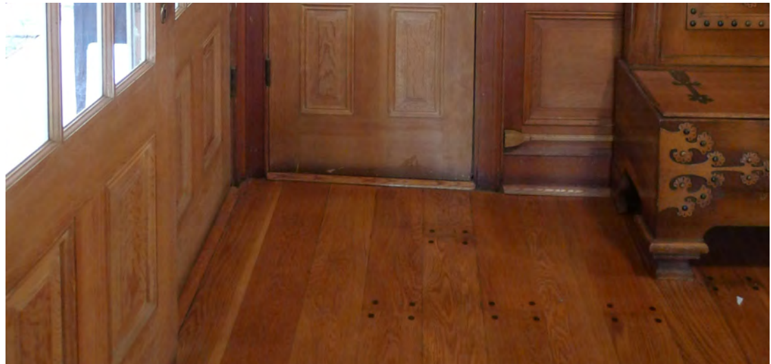
Figure 93. Oak floor with contrasting wood pegs in Room 101B.
