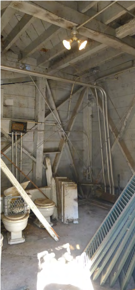
Figure 126. Room 101 - Tank House interior.
