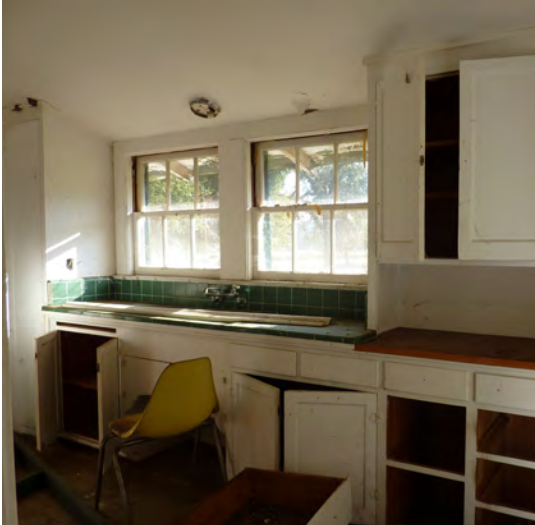
Figure 347. Cabinets in the Kitchen.
