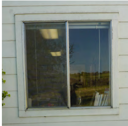
Figure 223. Non-contributing aluminum window at 1960s addition.
