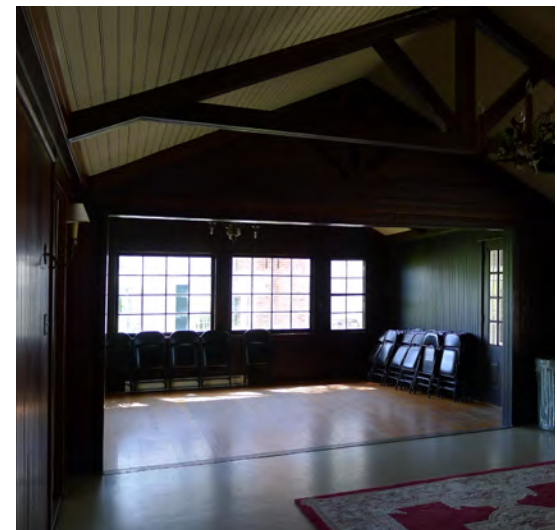
Figure 148. View of opening between Room 101 and 102.
