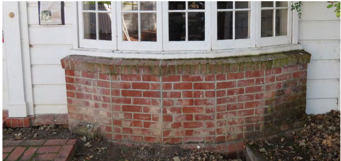
Figure 65. Brick cladding at Room 103 bow window.
