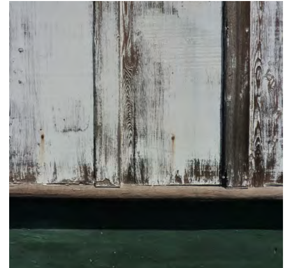
Figure 334. Paint deterioration.
