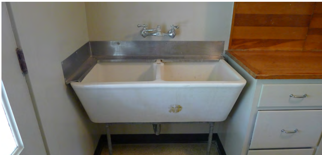
Figure 190. Original slop sink in Room 106.
