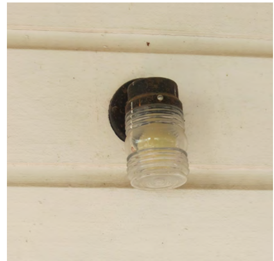
Figure 174. Sconce light fixture on southwest elevation.
