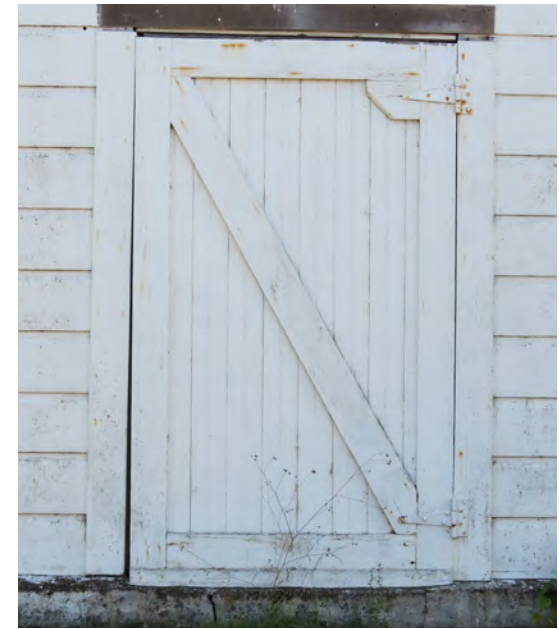
Figure 221. Frame-and-fill door at Room 119.
