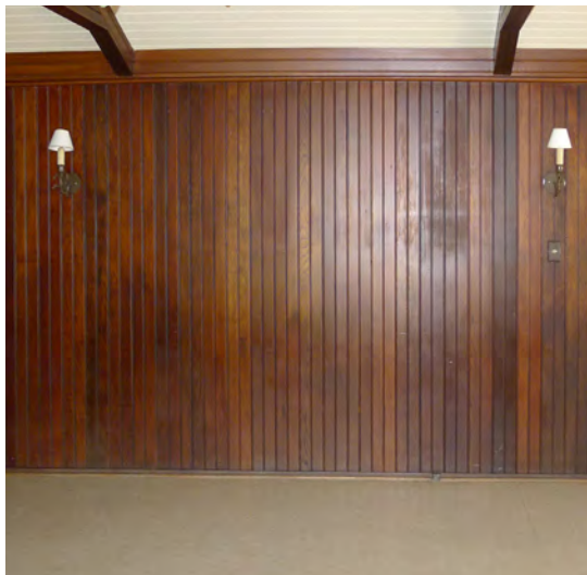
Figure 179. Bead board wall in Room 102.
