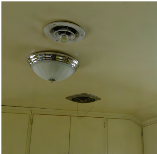
Figure 247. Painted gypsum board ceiling in Room 102 - Kitchen with various fittings.
