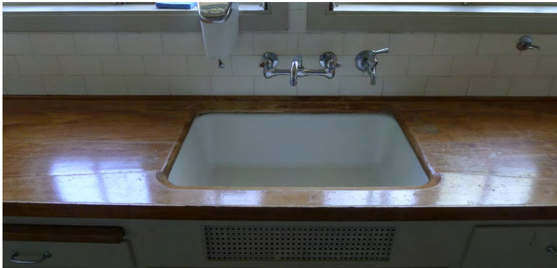
Figure 189. Original sink in Room 103.
