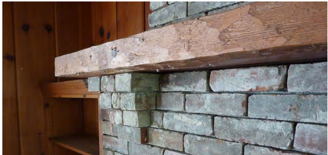
Figure 351. Wood mantel supported by a protruding brick corbel.
